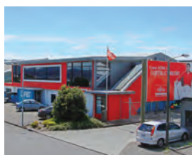
Fujitsu General New Zealand Ltd. (Nowa Zelandia)
